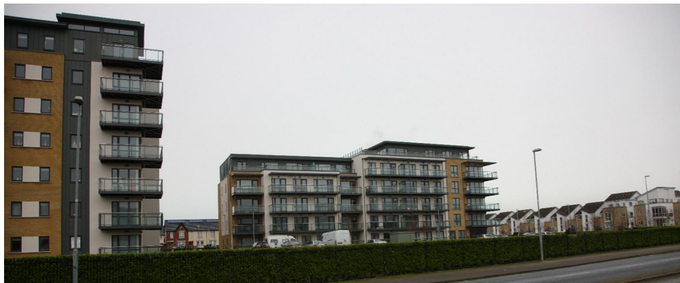
Figure 10.7: The Hermitage development near the site includes a seven storey apartment building
