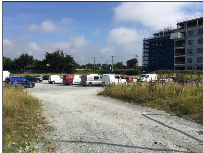
Plate 14.7 Temporary car park, facing north-northeast
