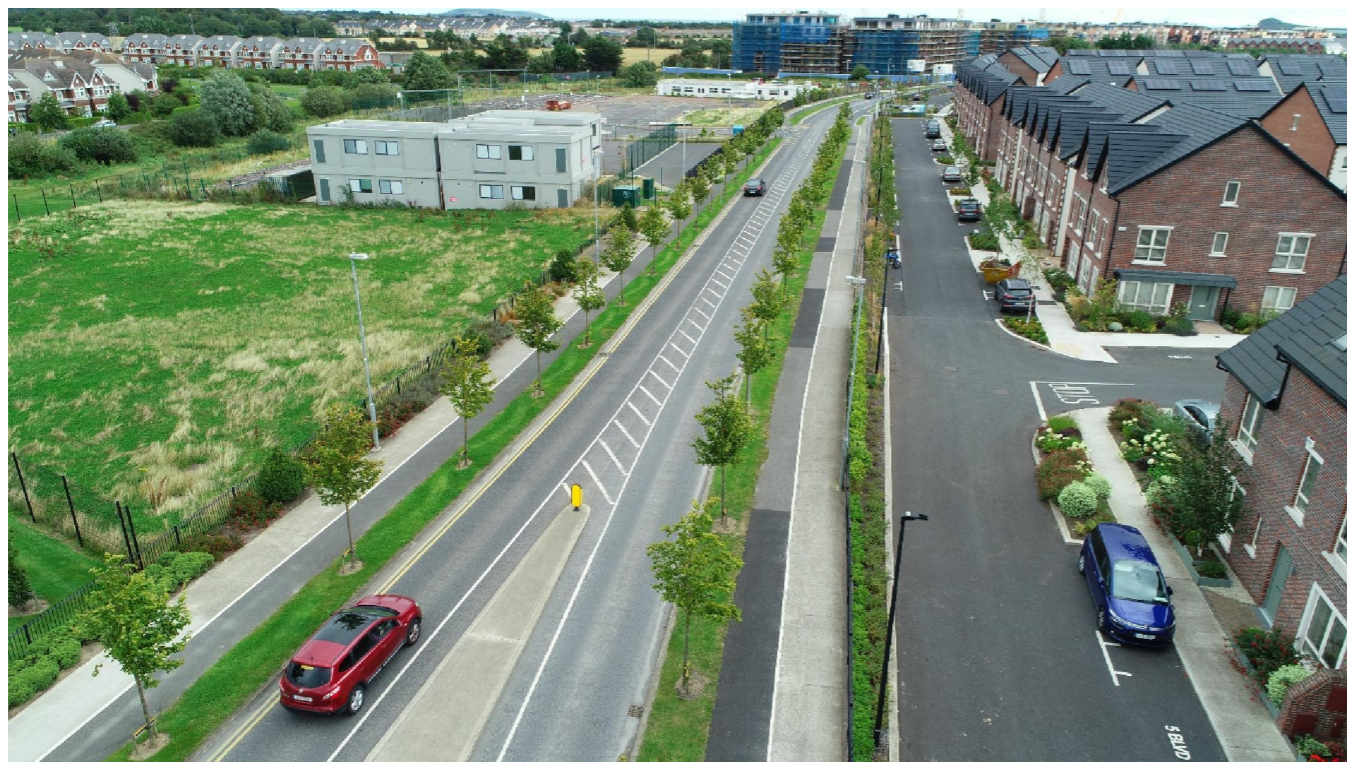
Figure 10.11: Bird's eye view from the south west corner of the site. Note the high density (six storey) development under construction to the east of the site across Balgriffin Park
